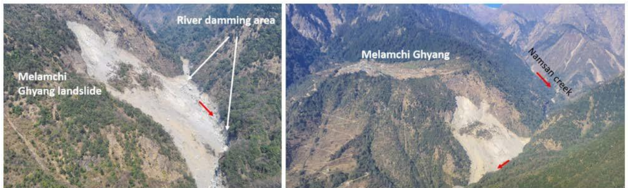
Figure 3-5. View of Melamchi Ghyang Area and landslides that caused landslide dam (Sources WB, 2021).
